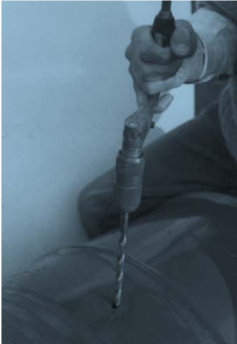
First, drill a hole of 6 mm and afterwards a hole of 16 mm into the marked spots
